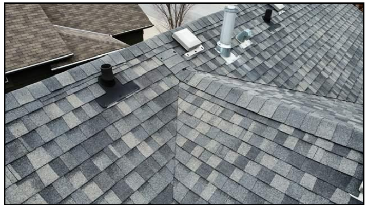
Asphalt shingles
