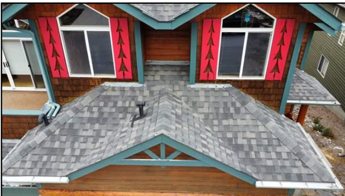
Asphalt shingles
