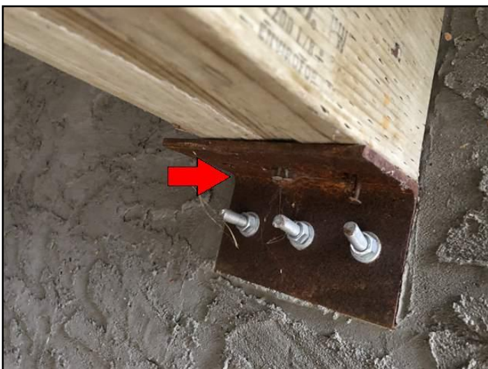
Fastener To Exterior Wall
