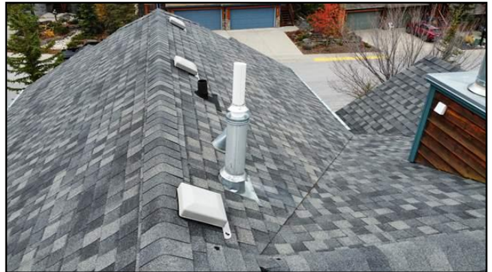
Asphalt shingles
