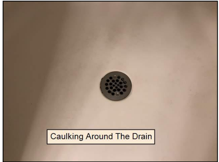
Caulking loose, missing or deteriorated
