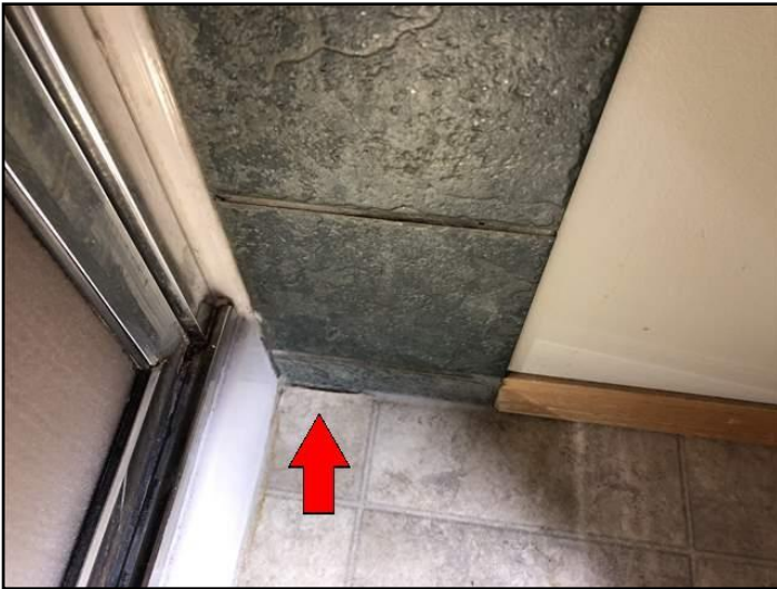
Caulking loose, missing or deteriorated
